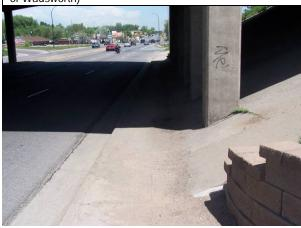
Missing curb ramp on northeast corner of 8th Place and Wadsworth
